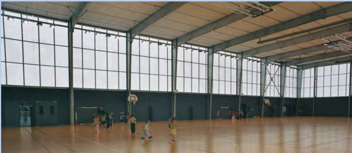
Sportshall Carquefou, France Architect Murail, Nantes 650 Lux right in the centre of the sportshall
