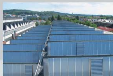
Mounted on a Northlight roof
