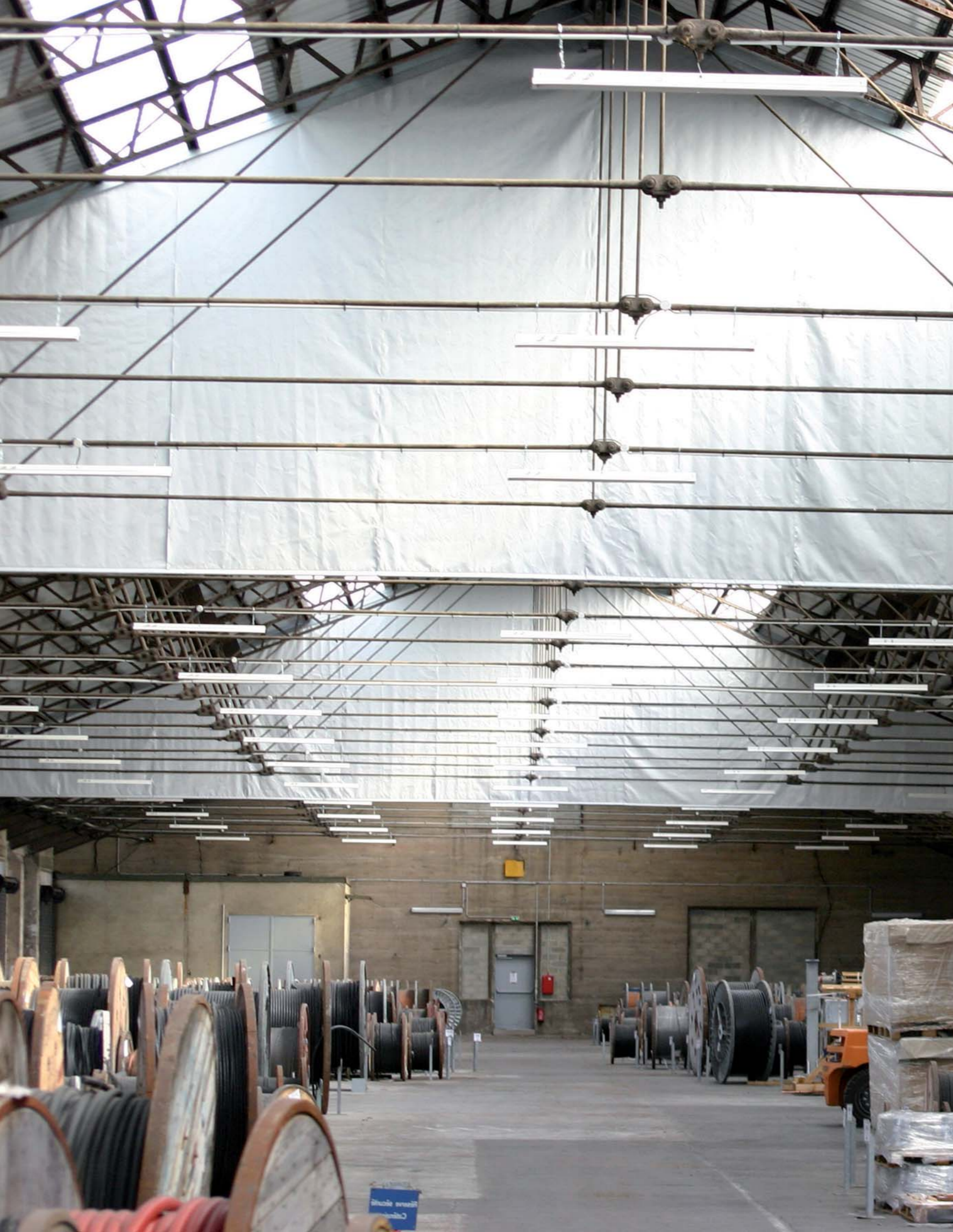
Picture: Static SmokeTex smoke curtain that has been adapted to the slope of the roof
