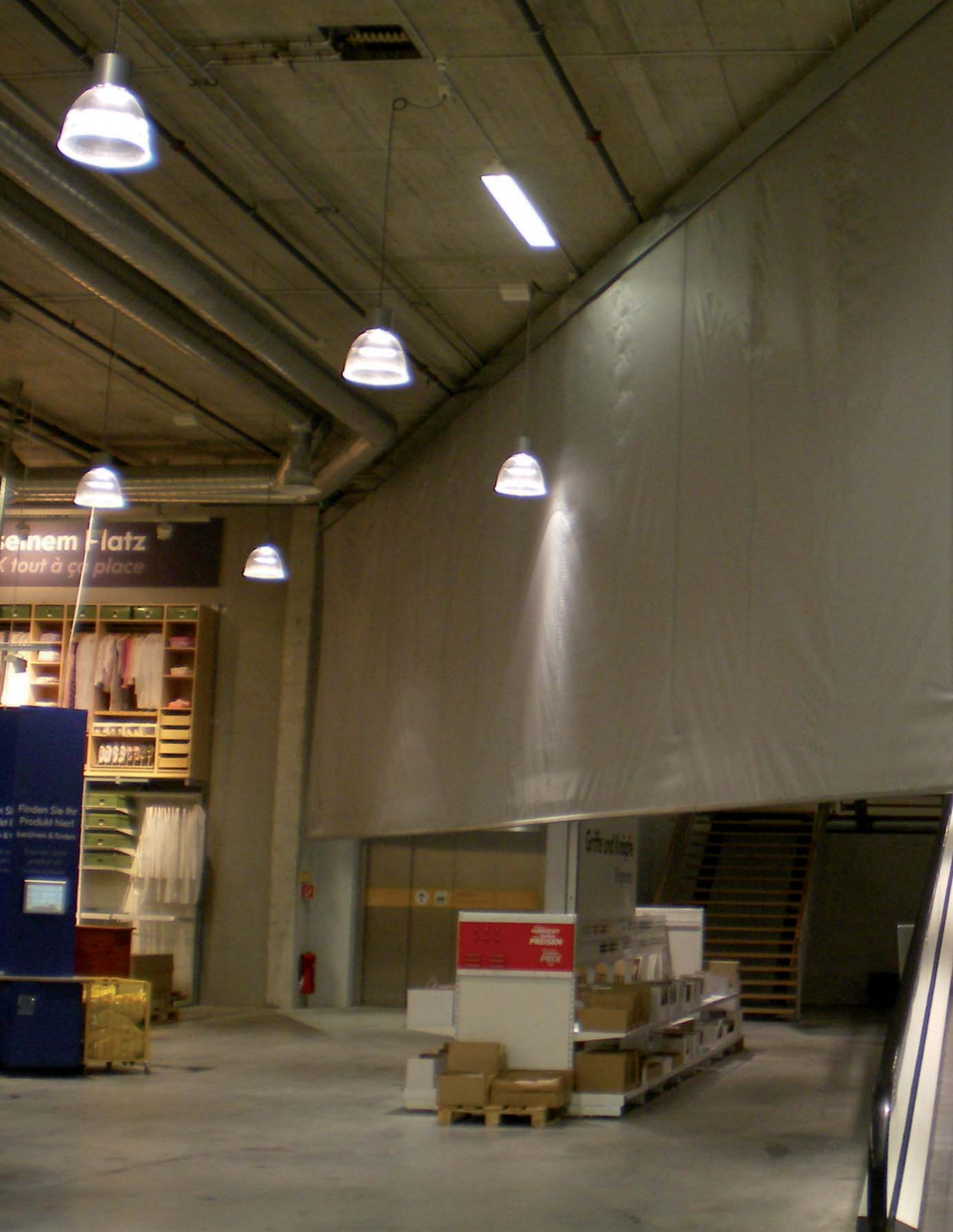
Picture: In the event of a fire, the rolled smoke curtain drops down in order to keep the stairs free of smoke
