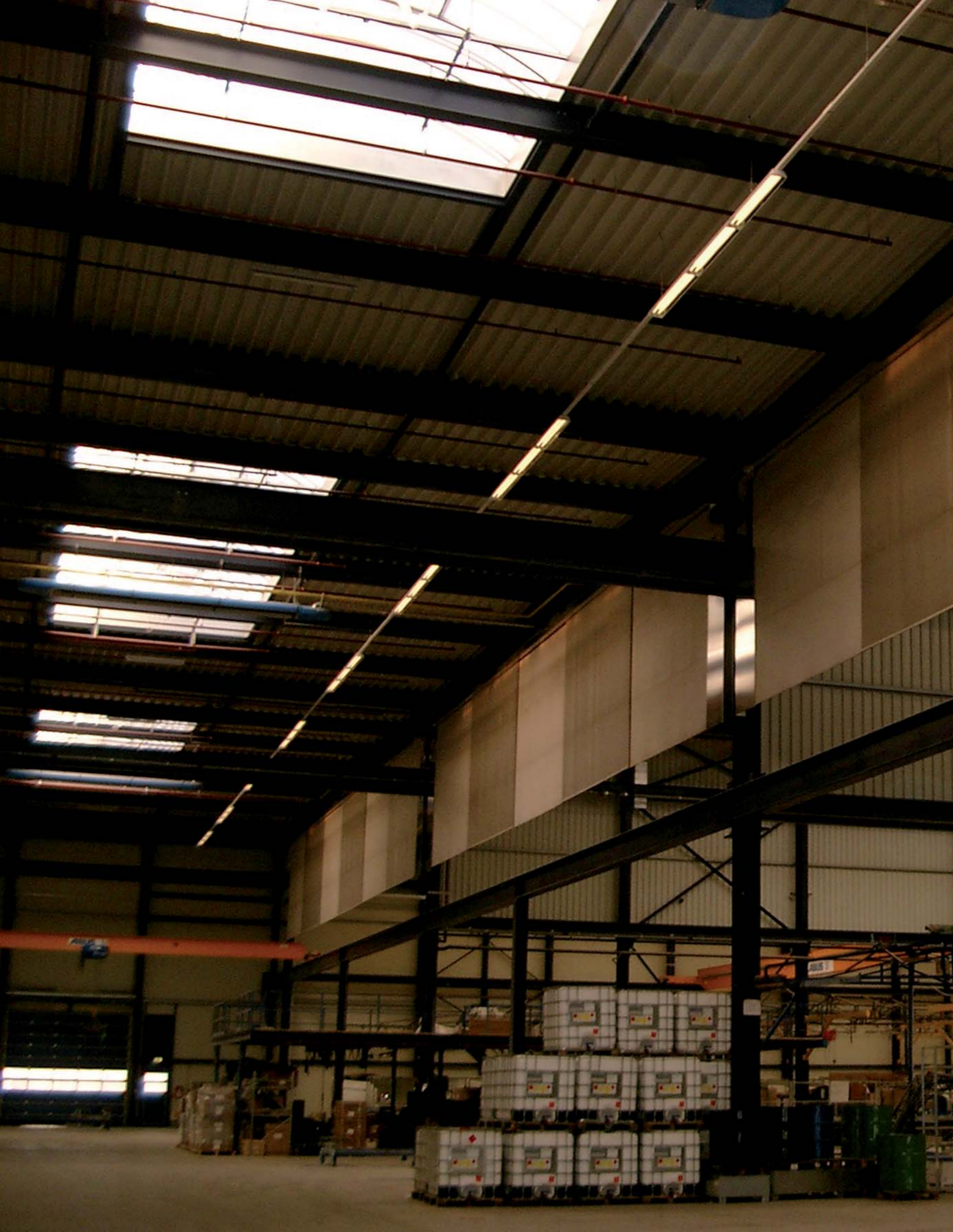
Picture: Rigid smoke curtains above a crane runway
