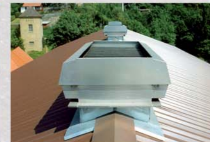
On a gable roof ridge
