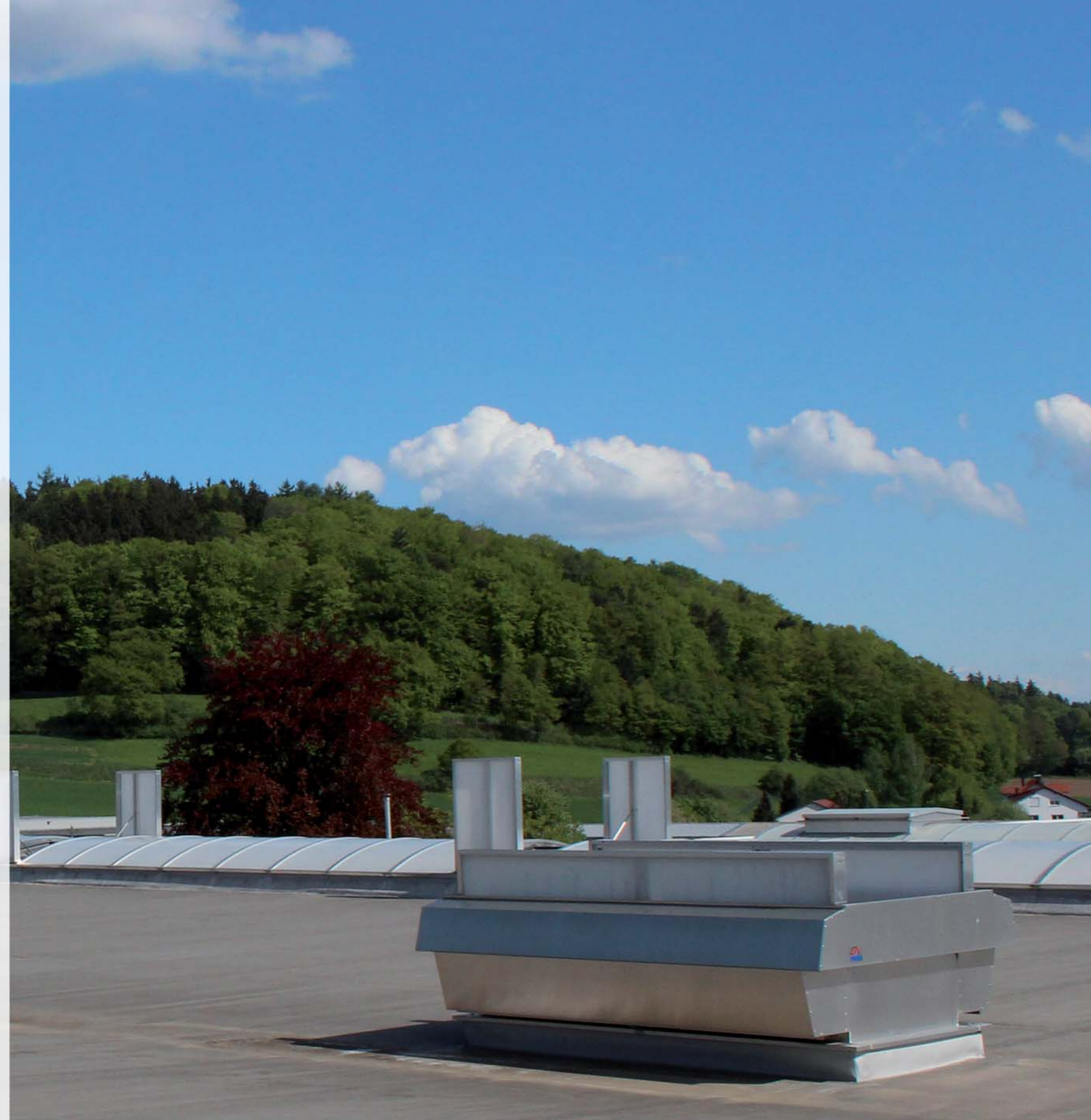
Large illustration: MEGAPHOENIX as a stand-alone unit on a factory building.
