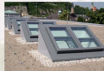
Mounted on a sloped plinth
