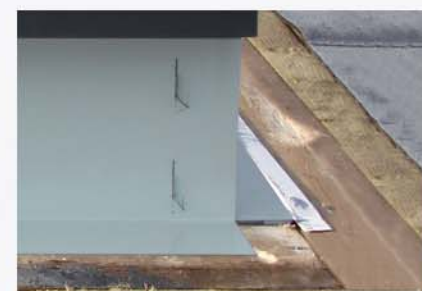
Plug-in plinth before gluing-in
