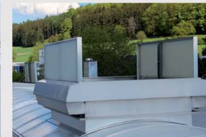
MEGAPHOENIX on a skylight
