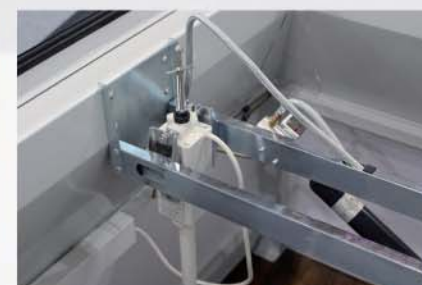
Separate drive for daily ventilation
