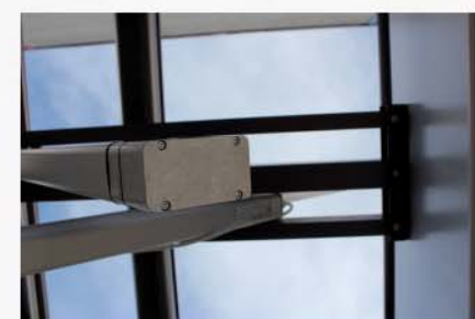
90° opening panel position for ventilation
