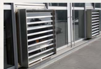
SMOKEJET in vertical glazing
