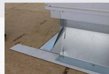
Plug-in plinth before gluing-in
