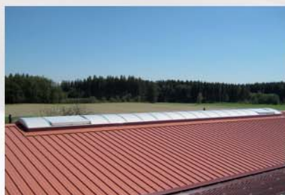
On top of a saddle roof ridge
