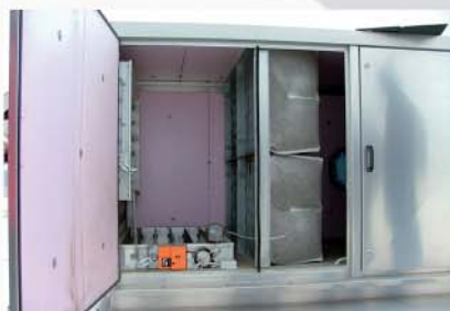
Mixed-air unit and bag filter
