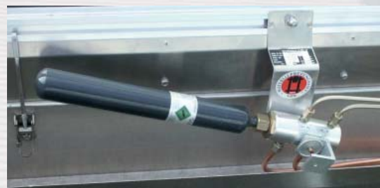
thermal priority valve connected to a CO 2 cartridge
