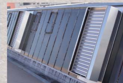
MULTIJETs in a Northlight roof
