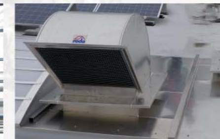
Roof-mounted suction hood
