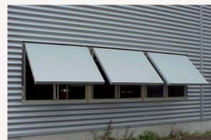
PHOENIX as a wall-mounted air-supply unit
