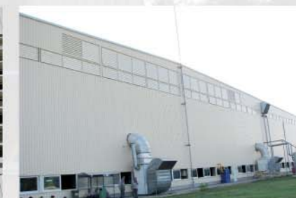
AIRJET mounted in a wall
