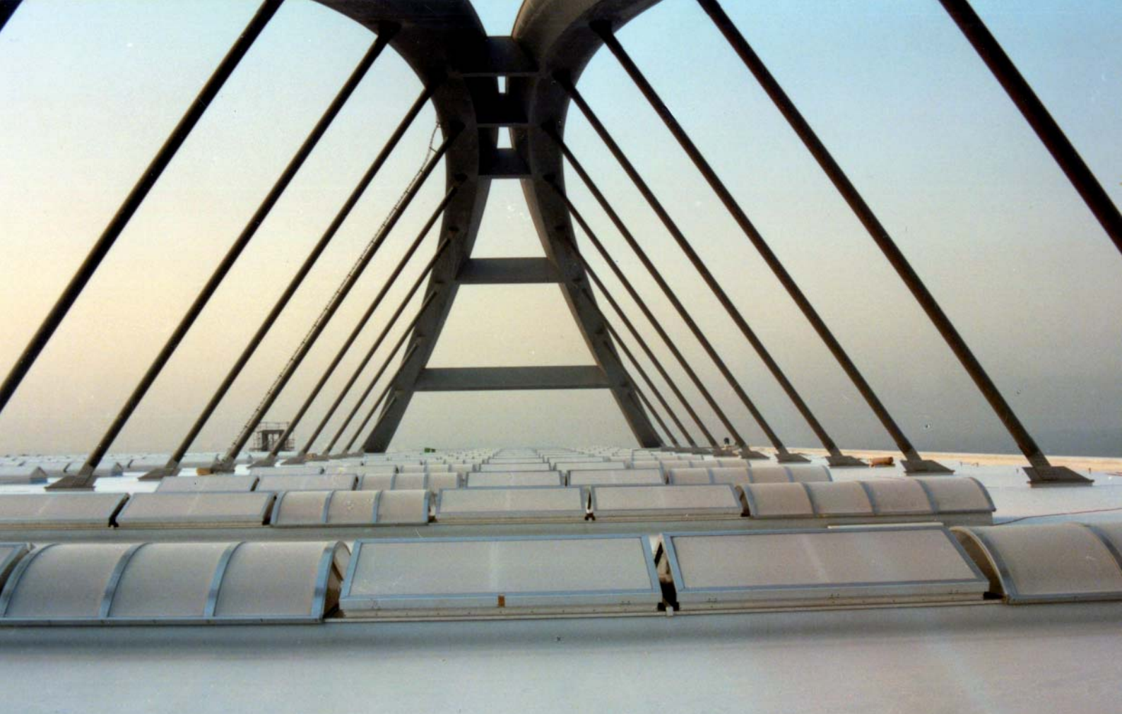
This picture was taken back in 1991 after the installation.
