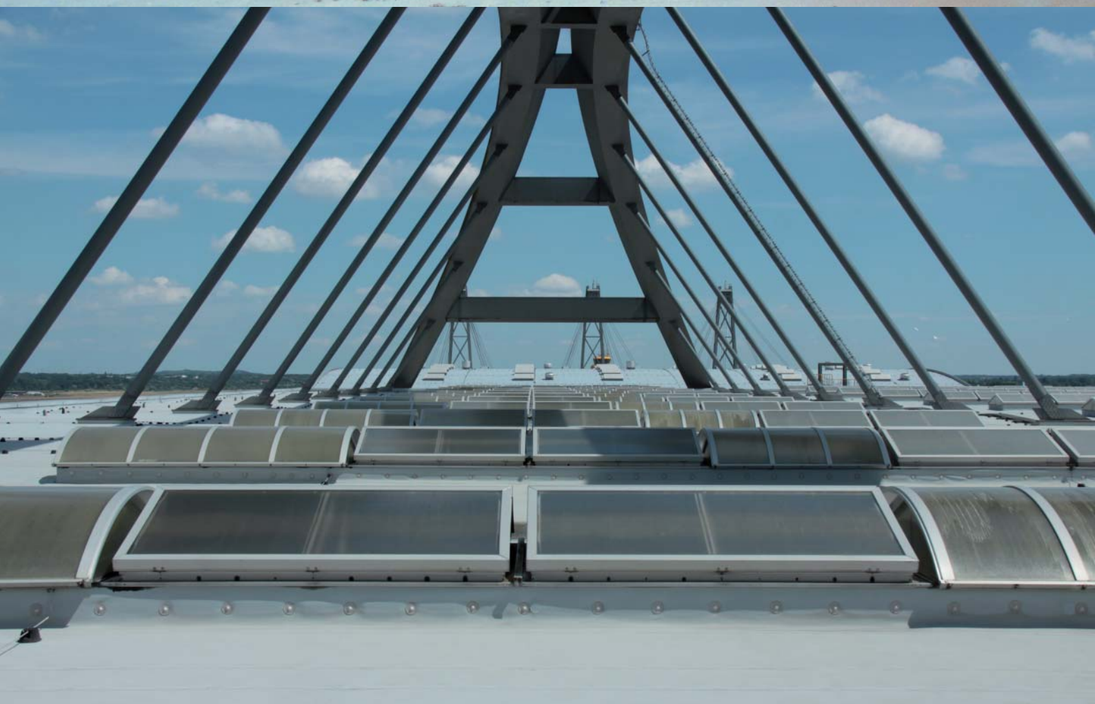
25 years later, the multiwall panels have yellowed and allow considerably less sunlight to enter the building.
