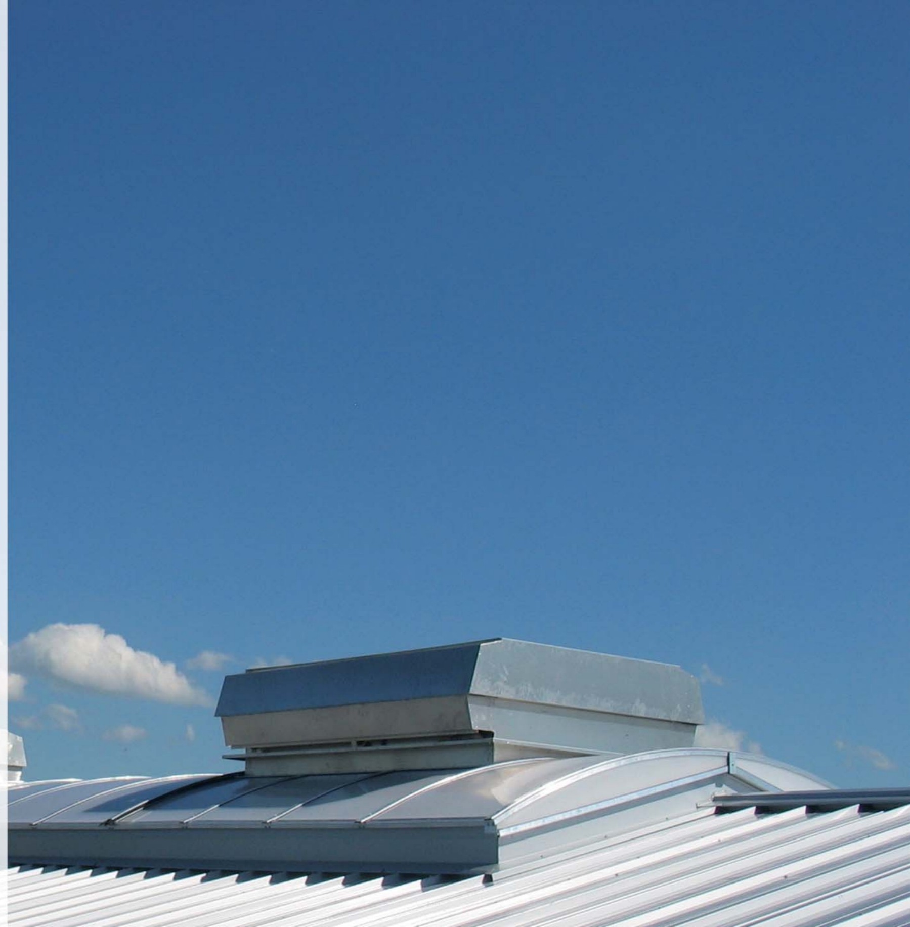
The SHE and ventilation systems may also be integrated into a continuous skylight system, which allows daylight to enter the building and thus decreases operating
