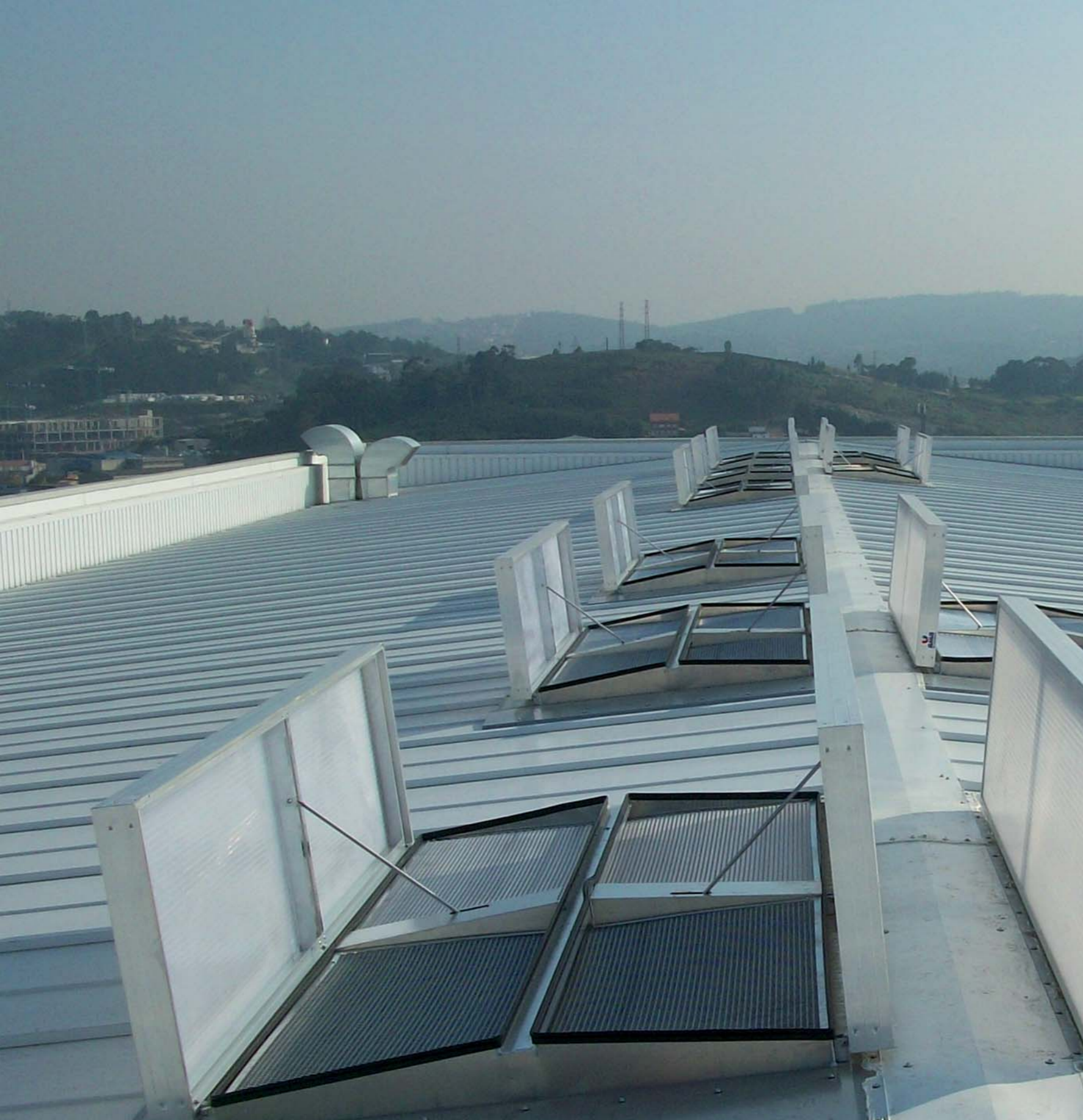
PHOENIX SHE and ventilation systems fitted with insect screens
